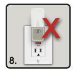
Malfunctioning GFCIs <u>do not</u> provide shock protection. Have a licensed, qualified electrician check the GFCI and correct the problem if your GFCI is not working.
